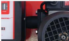
Connection of the meter to the pump through a long flange.
